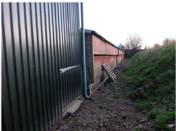
Excavated bank to rear of original Buildings
