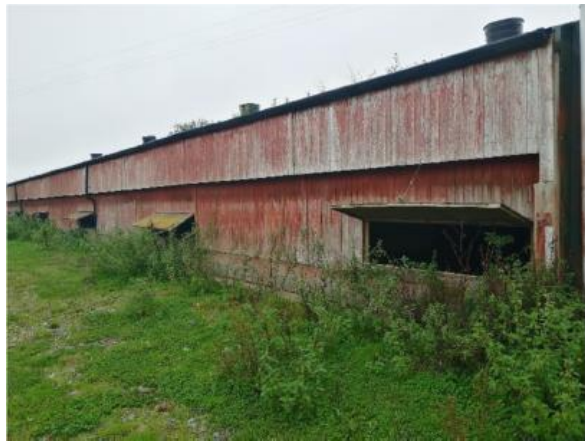
Eastern elevation of original building
