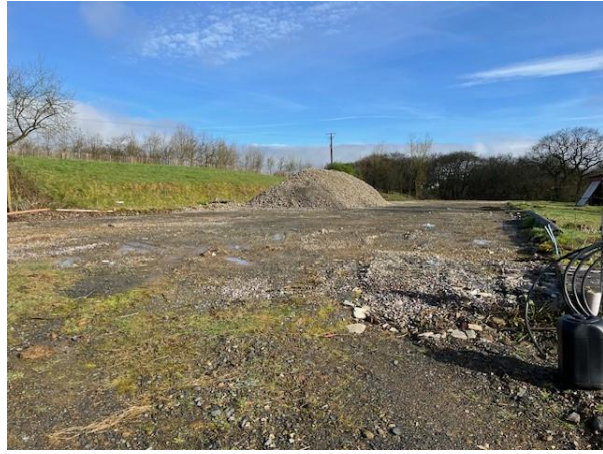
Buildings have now been demolished
