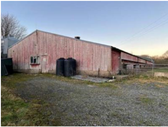
Gable end of original building facing northwards
