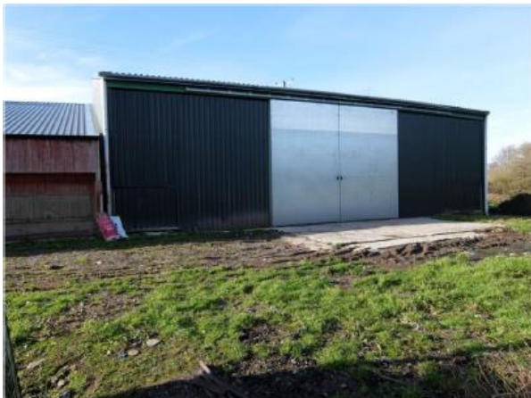
Eastern elevation of original taller steel portal framed addition
