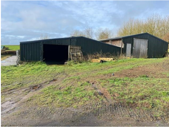
Buildings to south of site
