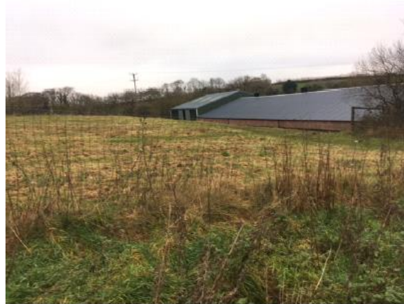
Original buildings when viewed from the west
